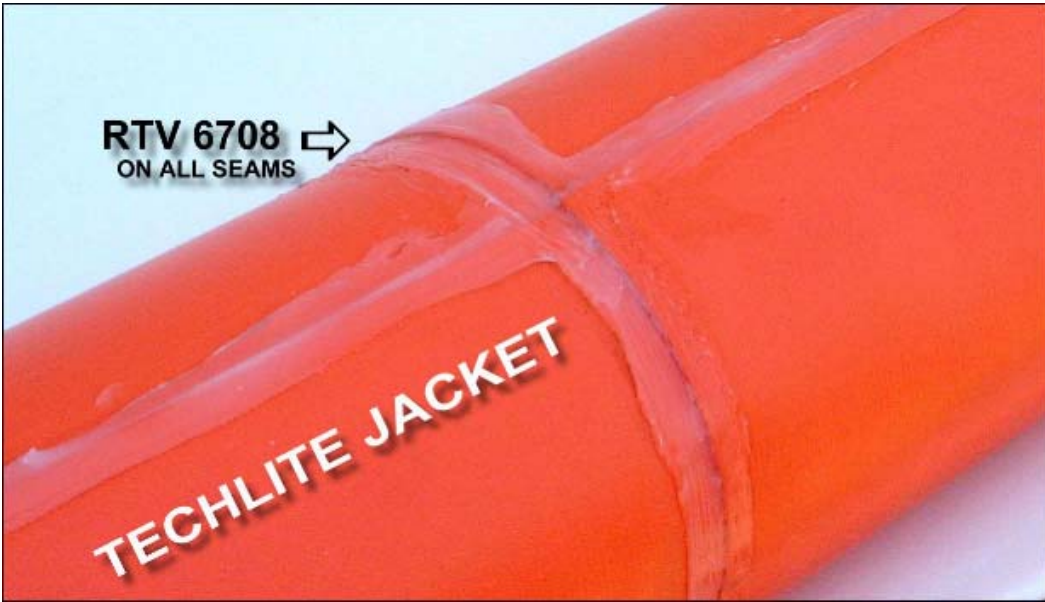
Photo # 1 All seams over sealed with RTV
